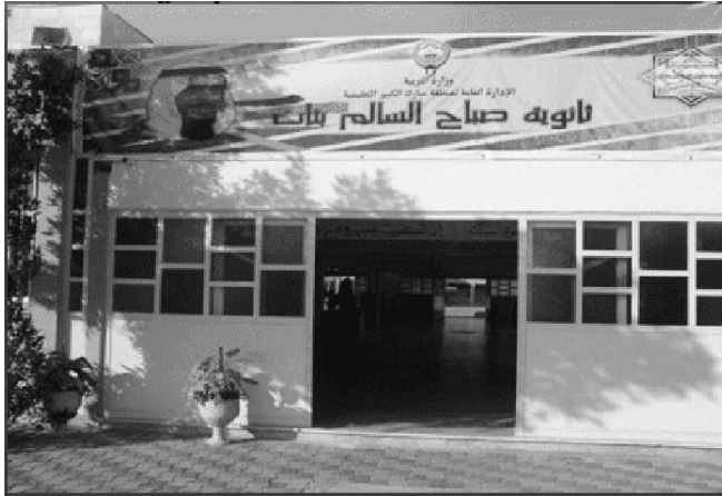
FIGURE 1 the schools of Kuwait designed to resist its harsh summer climate (Source: www.moe.edu.kw )
