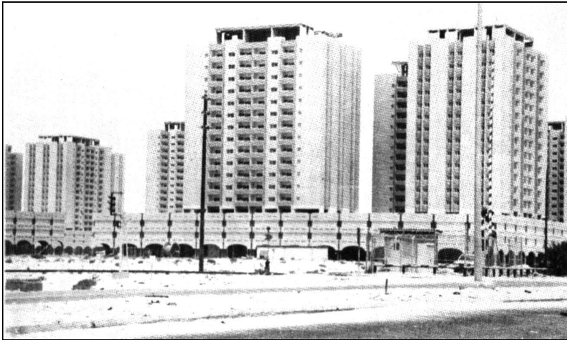
Fig. 1- Typical high rise apartment buildings constructed in the major cities of Saudi Arabia. The conception, design and structure of these housing projects, based on imported concepts and different cultural values
